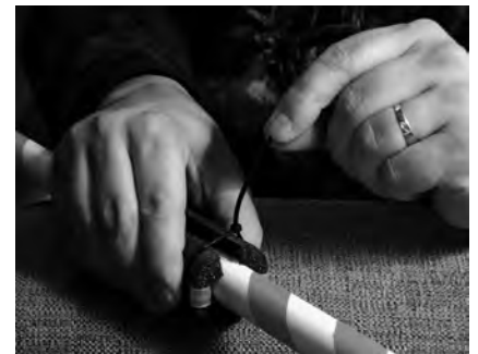
Securing the pipe foam with zip ties
